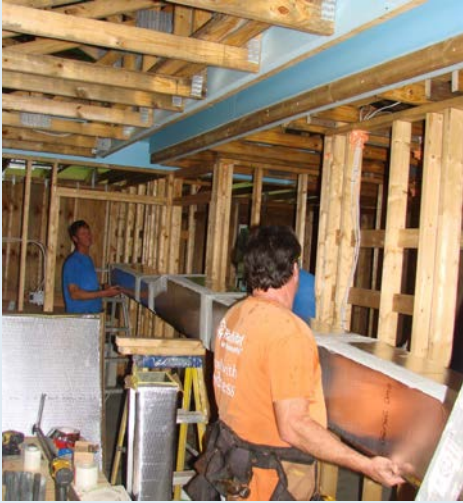
Main duct is lifted into place.
