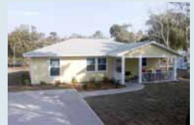
Southeast Volusia HFH homes feature ENERGY STAR® windows, equipment, fixtures, and appliances
