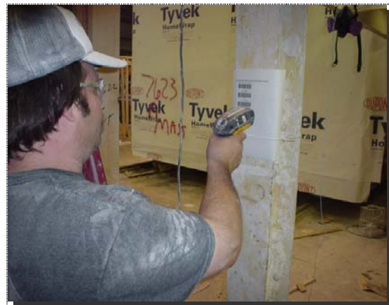
Figure 26 Scanning drywall activities with new STACs device.
