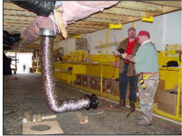
Figure 27 Southern Energy Homes quality control engineer conducts in-plant duct leakage test.
