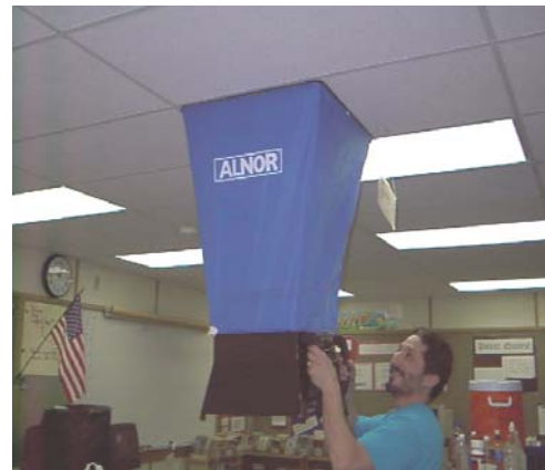
Figure 54 Ventilation system testing at North Thurston School District.
