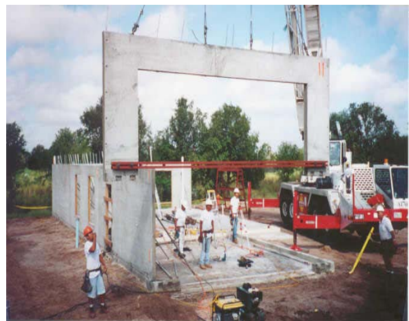
Figure 2 Setting pre-cast concrete wall panel
