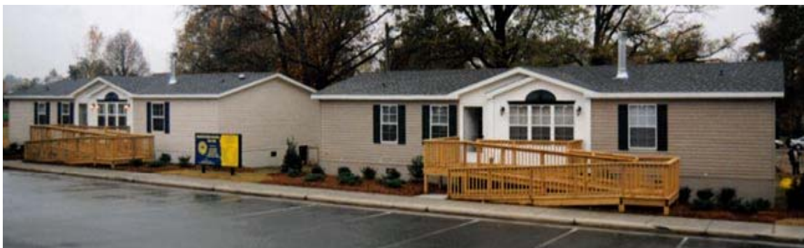
Figure 50 Side-by-side monitoring of manufactured homes at NCA&TSU.
