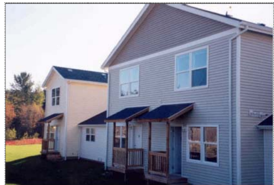
Figure 22 Nogi Gardens, America's first HUD Code attached town houses.
