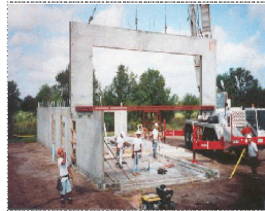
Figure 30 Setting pre-cast concrete wall panel.
