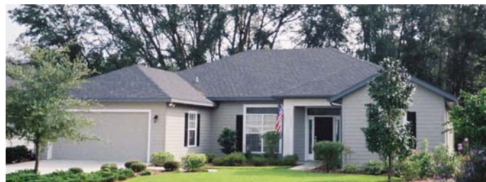
Figure 5 Atlantic Design and Construction home in the Mentone neighborhood.
