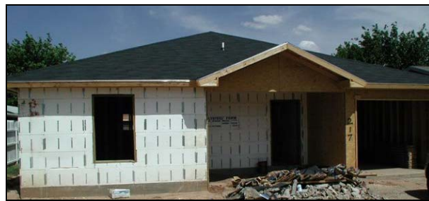
Figure 10 Low income housing built by the City of Lubbock using insulated concrete forms.
