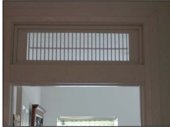
Figure 18 Transom return air pathway with operable louvers blends in with the vernacular aesthetics of this DESIGNhabitat Energy Star home built in conjunction with Auburn University’s College of Architecture.
