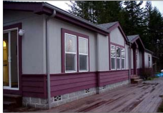
Figure 45 WSU Energy House in Olympia, WA
