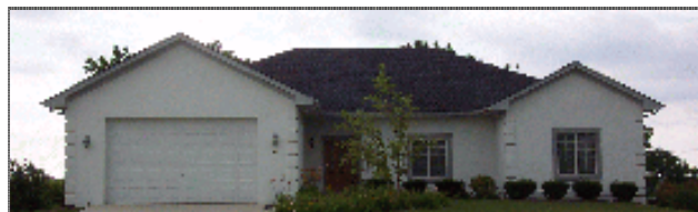
Figure 11 Completed Dukane Precast home tested by BAIHP
