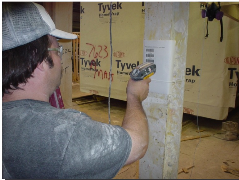
Figure 4. Scanning drywall activities at Avis America
