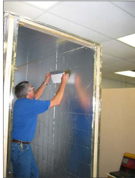
Figure 81 Installing unbaffled return air flow through wall grille
