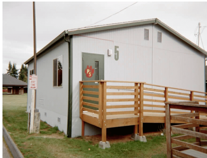
Figure 52 64 Energy efficient portable classroom at Pinewood Elementary School in Marysville, Washington
