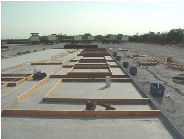
Figure 1 Panel forms on forming bed
