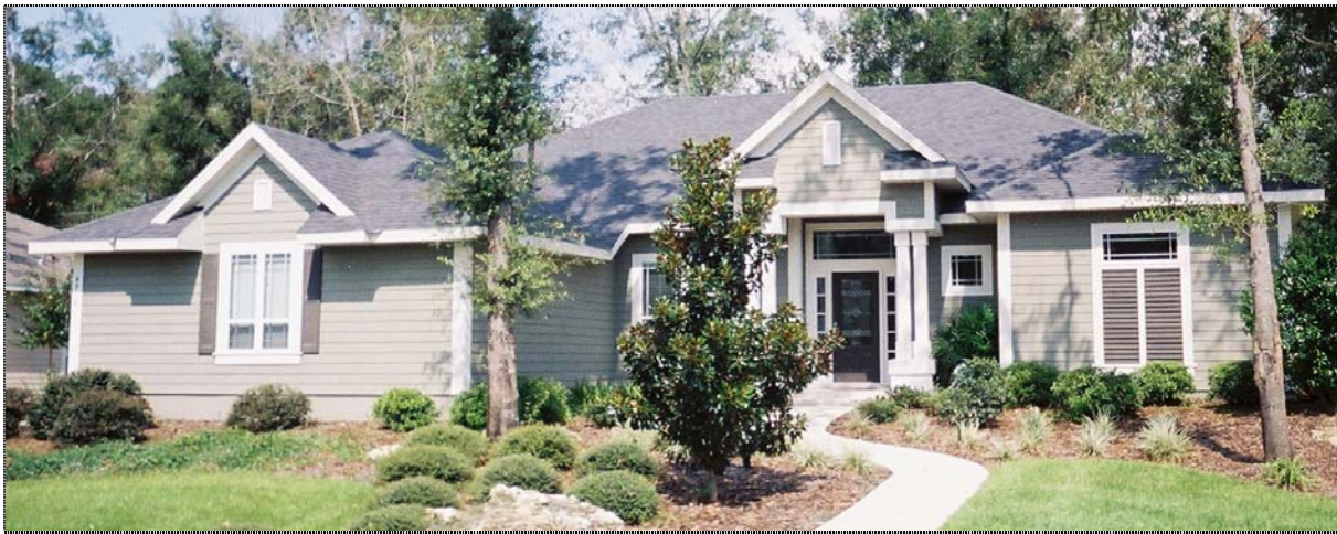
Figure 2 Building America homes like this one built by BAIHP Industry Partner G.W. Robinson Homes in the Cobblefield community (Gainesville, Florida) reduce energy bills for individual homeowners while pushing the standard of building closer to DOE's 2010 goals.
