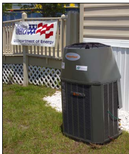
Figure 70 Final test prototype with diffuser and fan.
