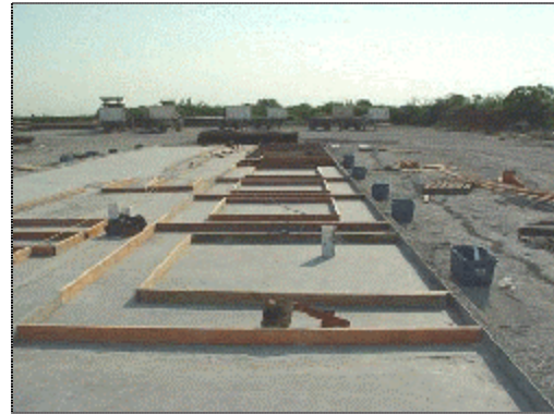
Figure 29 Panel forms on forming bed.
