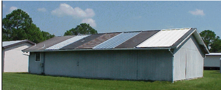
Figure 87 Flexible Roof Facility in summer of 2003 configuration.
