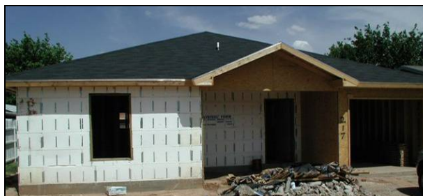
Figure 12 Low income housing built by the City of Lubbock using insulated concrete forms.
