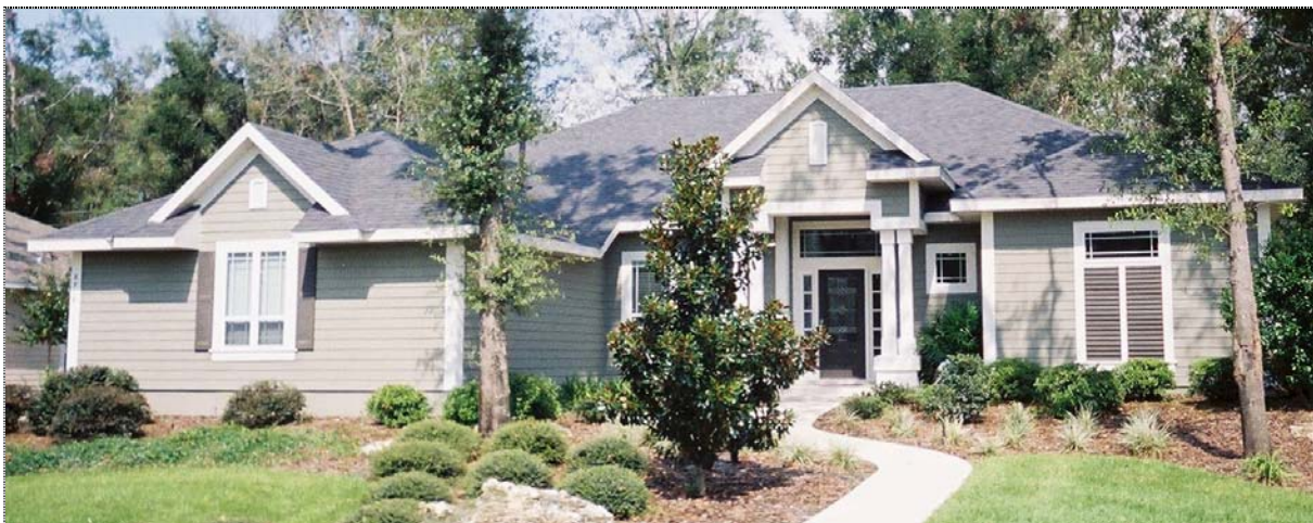
Figure 2 Building America homes like this one built by BAIHP Industry Partner G.W. Robinson Homes in the Cobblefield community (Gainesville, Florida) reduce energy bills for individual homeowners while pushing the standard of building closer to DOE’s 2010 goals saving 30% in whole house energy use (source energy) compared to the 2005 Building America benchmark.
