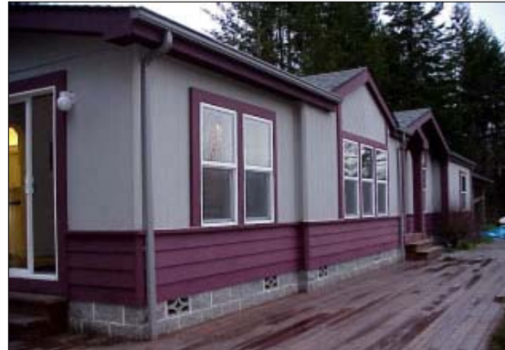
Figure 56 WSU Energy House in Olympia, WA
