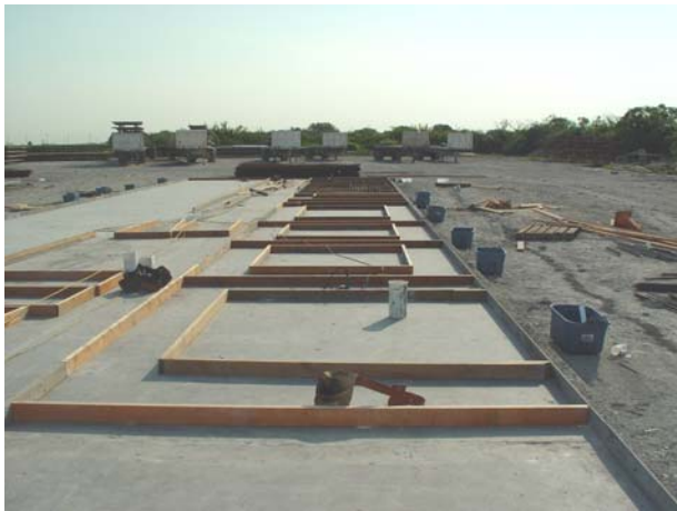
Figure 1 Panel forms on forming bed
