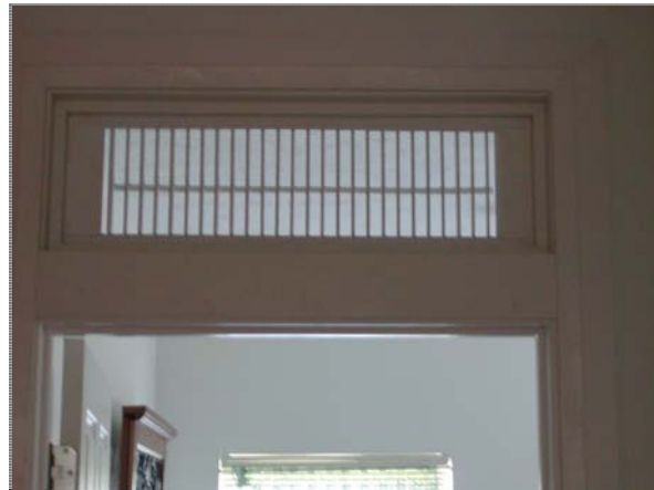
Figure 24 Transom return air pathway with operable louvers blends in with the vernacular aesthetics of this DESIGNhabitat Energy Star home built in conjunction with Auburn University's College of Architecture.
