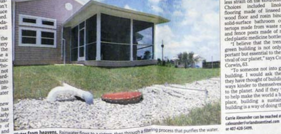
Water from heavens. Rainwater flows to a cistern, then through a filtering process that purifies the water.
