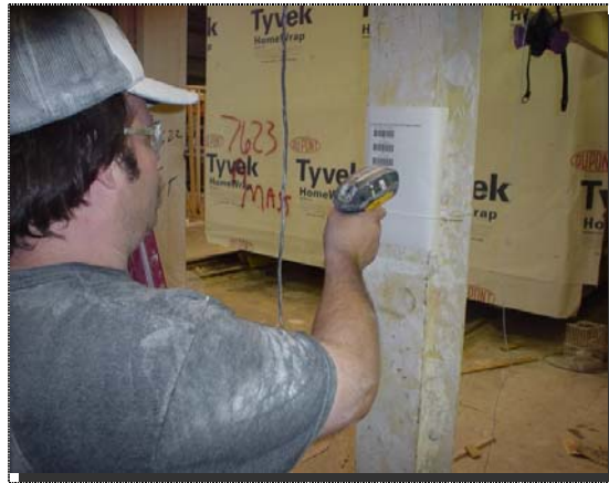
Figure 38 Scanning drywall activities with new STACs device.
