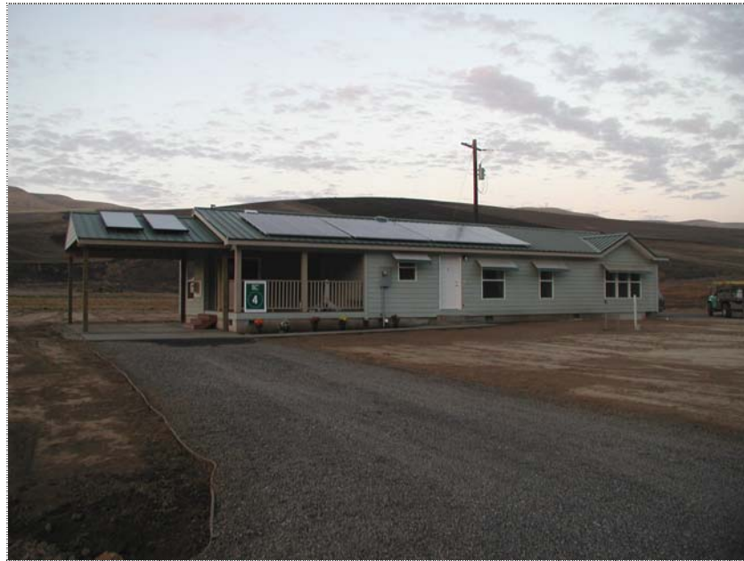
Figure 2 Zero Energy Manufactured Home, on site at the Nez Perce Fish Hatchery
