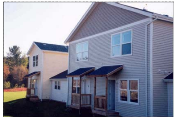
Figure 30 Nogi Gardens, America's first HUD Code attached town houses.
