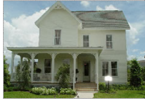
Figure 69 The Augusta, Cambridge Homes Building America Prototype.
