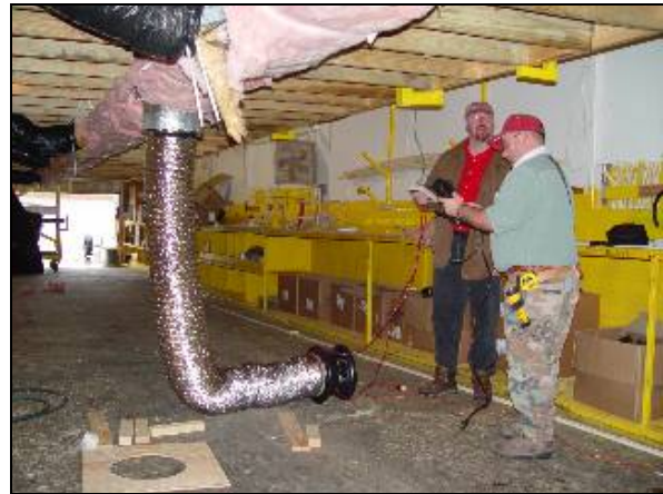
Figure 39 Southern Energy Homes quality control engineer conducts in-plant duct leakage test.
