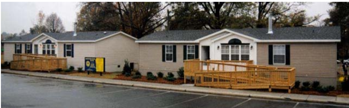
Figure 62 Side-by-side monitoring of manufactured homes at NCA&TSU.
