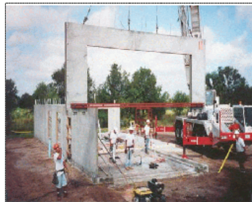
Figure 41 Setting pre-cast concrete wall panel.
