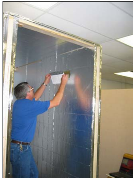
Figure 97 Installing un baffled return air flow through wall grille
