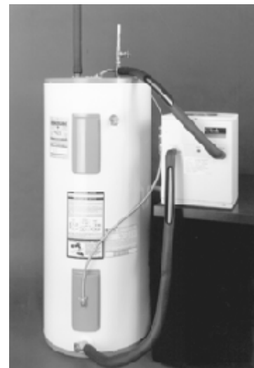
Figure 74 Heat pump water heater
