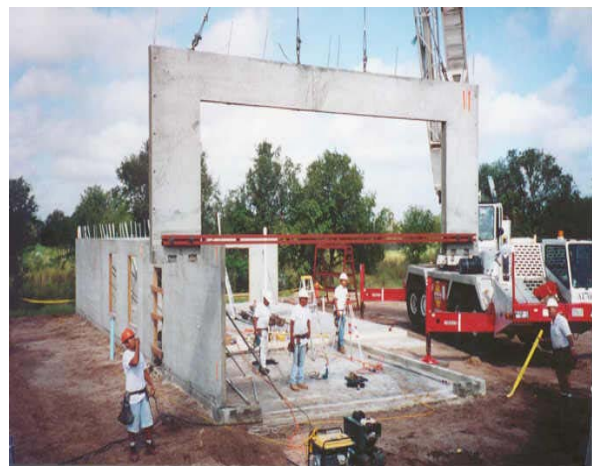
Figure 2 Setting pre-cast concrete wall panel
