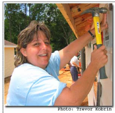
Figure 21 Homeowner Sandy Sedano installs rigid insulation (part of the energy package) on her new home during the 2003 JCWP at the Anniston (AL) site.
