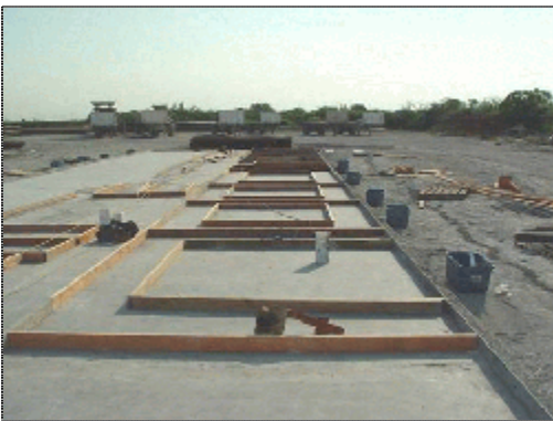
Figure 40 Panel forms on forming bed.
