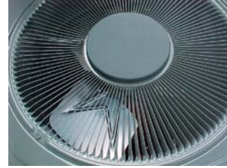
Figure 83 Air conditioning condenser fan and diffuser.
