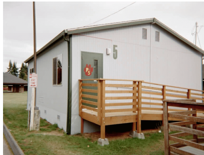
Figure 64 64 Energy efficient portable classroom at Pinewood Elementary School in Marysville, Washington
