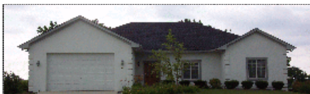
Figure 13 Completed Dukane Precast home tested by BAIHP
