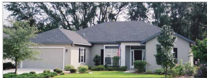
Figure 5 Atlantic Design and Construction home in the Mentone neighborhood.
