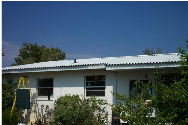
Figure 5 Finished light colored composite roof panels installed
