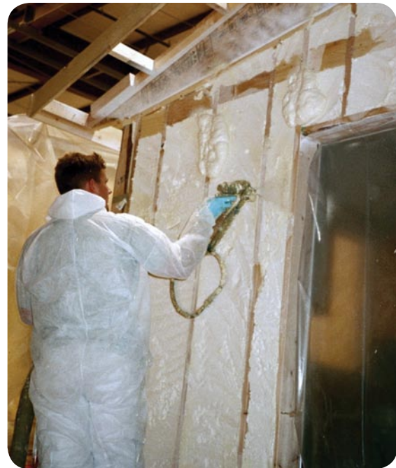
Icynene floor, ceiling, and wall spray-foam insulation resulted in the tightest HUD-code envelope and ducts ever tested.
